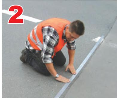
The edges of the surface to be repaired can be masked with "stone masking tape", to achieve clean edges (Fig. 2). The the surface to be repaired is lightly pre-wetted with a water brush to obtain better adhesion with the substrate (Fig. 3).
